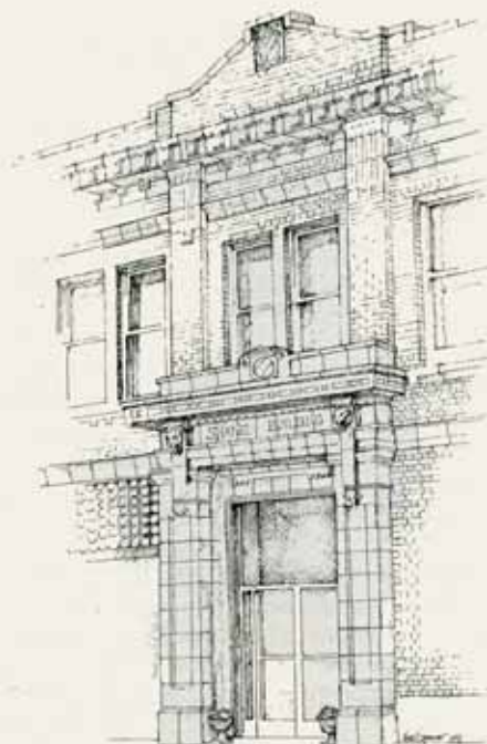
2 Shane Building (381 Shoup Avenue). This excellent example of the use of terra cotta with Renaissance Revival style was constructed in 1915. The main entrance of the building is surrounded by a terra cotta entablature with lion heads and a heraldic shield. Soon after it was built, the first floor housed a women's clothing store, a grocery store, and a furniture store.
